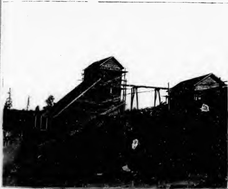
CHLORINATION PLANT OF SULTANA MINE.
